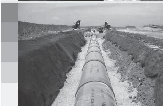
外圧管 External pressure pipes
