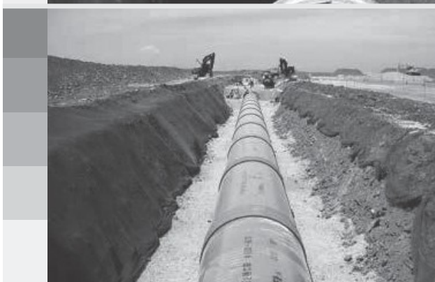
外圧管 External pressure pipes
